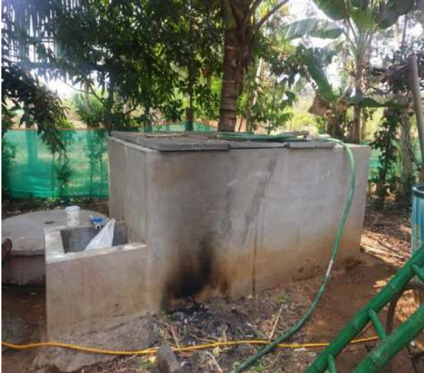
Tank to store the treated rain water
