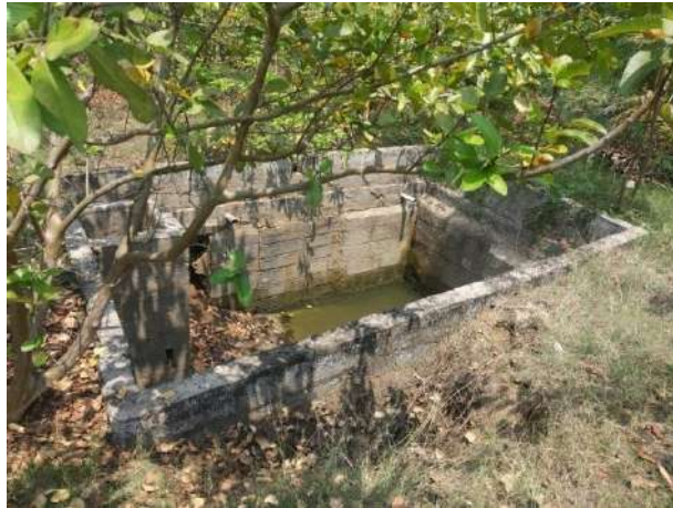
Artificial pit to store rain water
